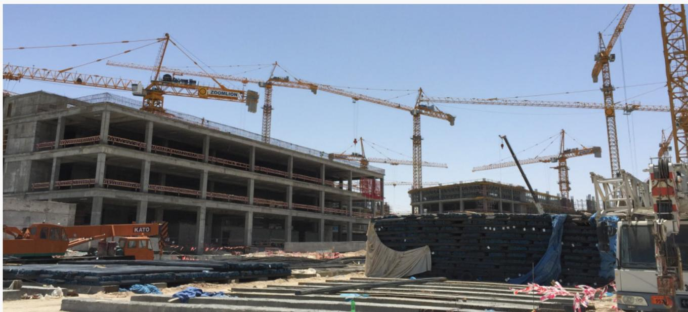
With a working radius of 70 meters, a height of 75 meters under the hook and a maximum capability of 7.8t at jib head, D800-42 has been especially configured for severe weather conditions and is therefore ideal for this project. A variable-frequency drive system was applied to hoisting, slewing and trolleying mechanism of cranes to ensure reliable control and steady movement. Besides an eddy current auxiliary controller configured in slewing system more enhanced the equipment stability.
